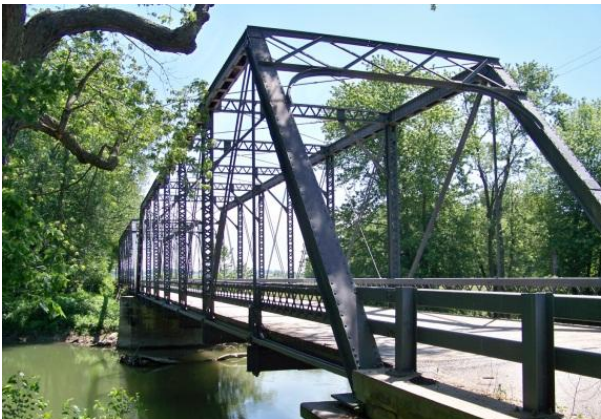
The Pugh Ford Bridge in Bartholomew County, Indiana built 1911 ↑
